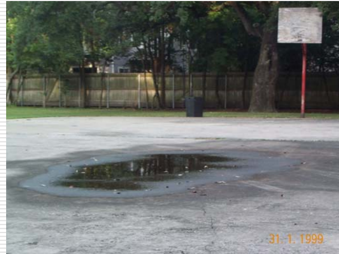
Deduct points for drainage
