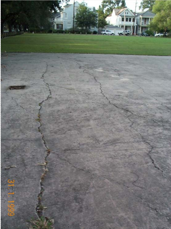
Deduct points for cracks
